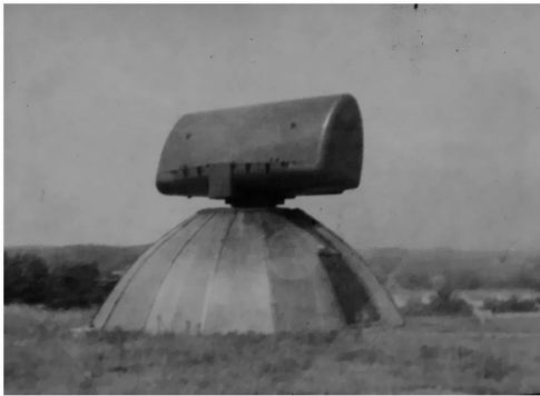
9 (Again, the Burlington installation)
