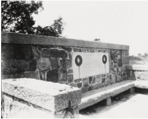
Here is the plaque, located on the bridge.
