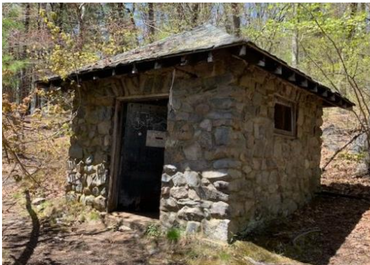
Pumphouse, built in 1913
